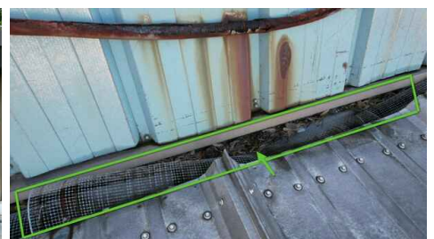
Roof Facade - Foam Used As Sealant - Example
