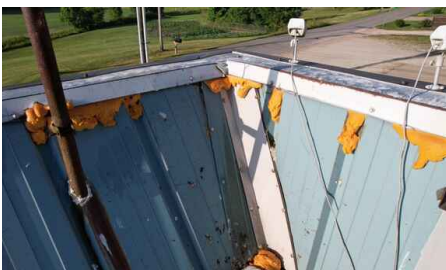
Roof Facade - Foam Used As Sealant - Example
