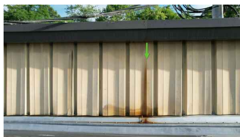
Roof Facade - Foam Used As Sealant - Example
