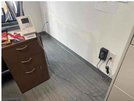
Front Left Corner Office, Area of Repairs
