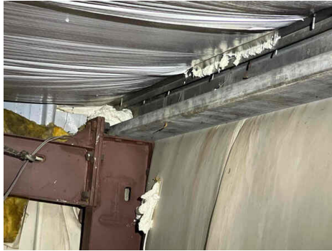
Above Ceiling Tiles - Spray Foam Used as Sealant
