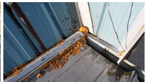
Roof Facade - Foam Used As Sealant - Example
