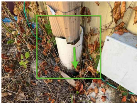
Left Side of Office, Downspout Partially Missing Underground Drain Pipe
