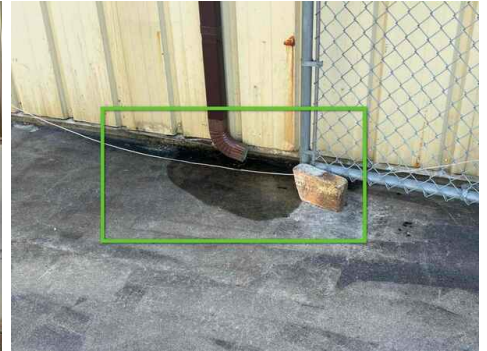
Left Side of Office, Downspout Drains Near Building
