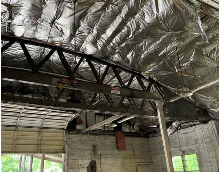
Interior Roof Structure
