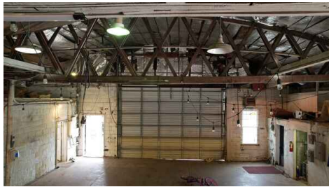
Interior Roof Structure
