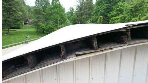
Front of Warehouse
