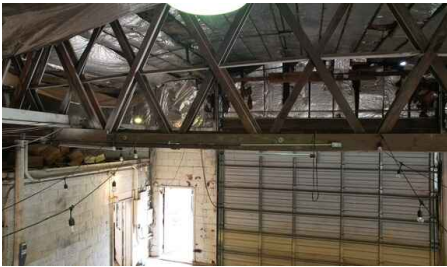
Interior Roof Structure
