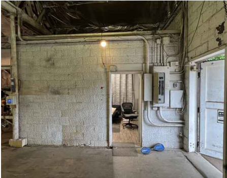
Main Warehouse Space
