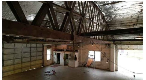
Interior Roof Structure
