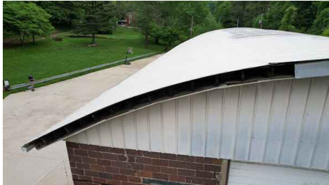
Front of Warehouse
