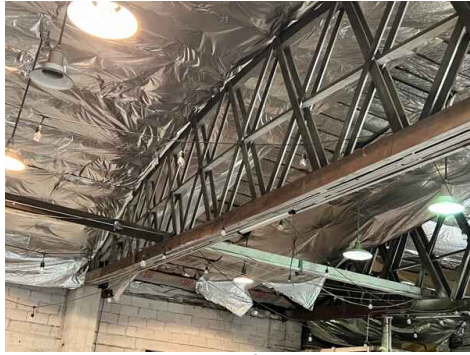
Interior Roof Structure
