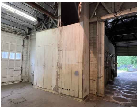
Main Warehouse Space
