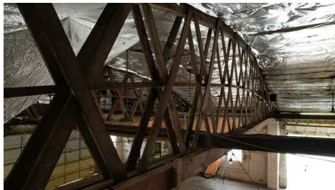
Interior Roof Structure
