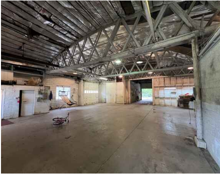
Main Warehouse Space
