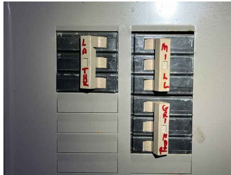
Main Warehouse Panels
