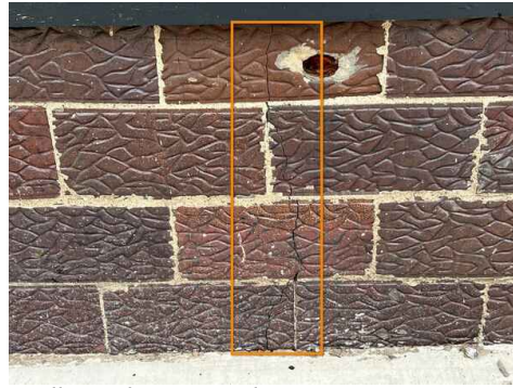
Wall Crack - Example
