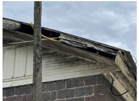
Rear of Warehouse
