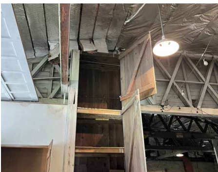
Main Warehouse Space
