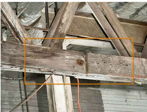
Rear Warehouse, Weekend Truss
