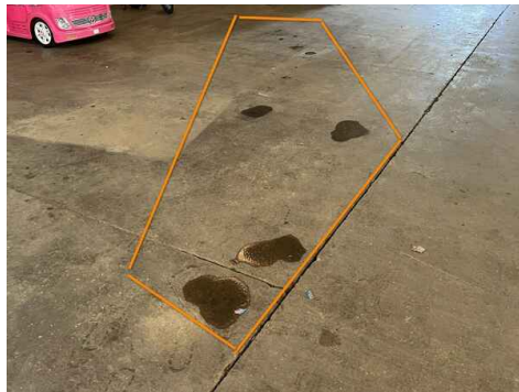
Example of Active Roof Leak Water Intrusion
