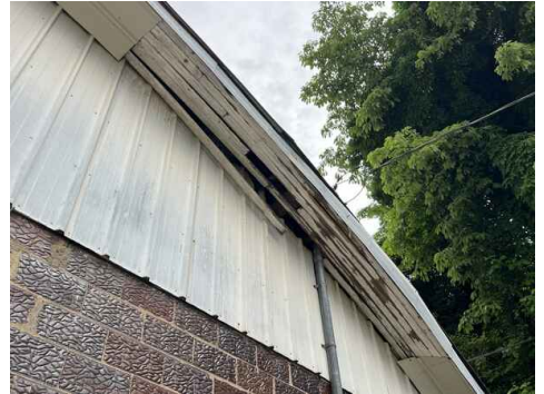
Front of Warehouse
