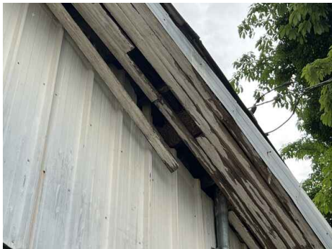
Front of Warehouse
