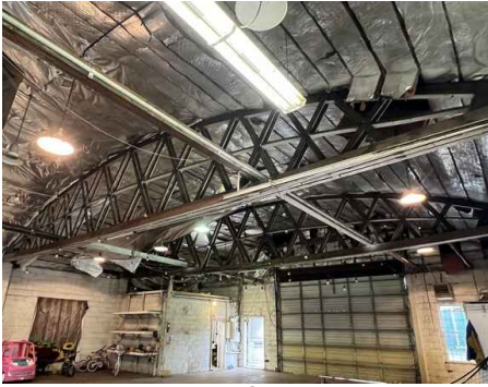
Interior Roof Structure
