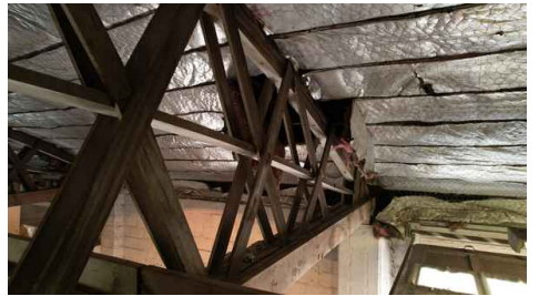
Interior Roof Structure
