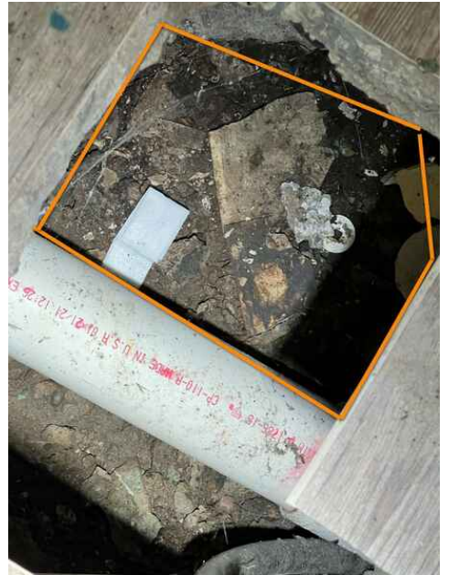
Below Bathroom Floor, Wet Soil
