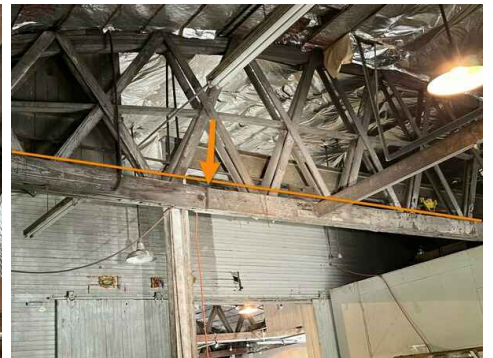
Rear Warehouse, Weekend Truss
