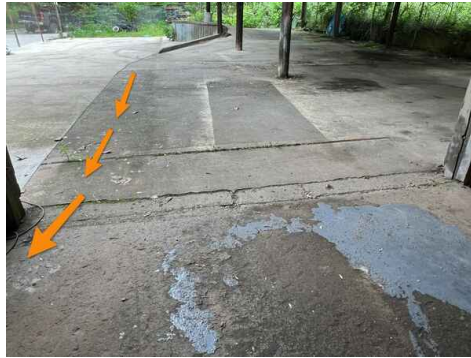
Example of Active Roof Leak Water Intrusion
