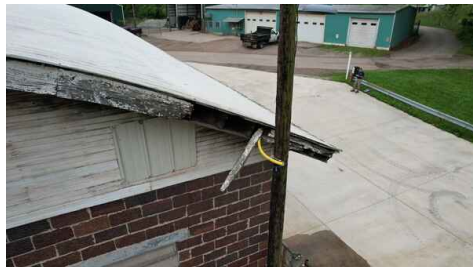
Rear of Warehouse
