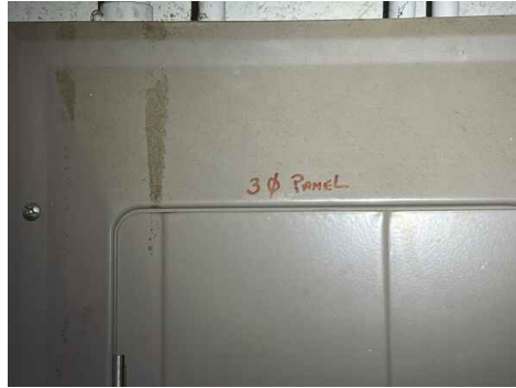
Main Warehouse Panels
