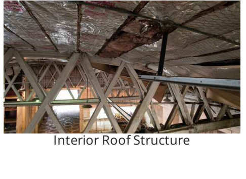
Interior Roof Structure
