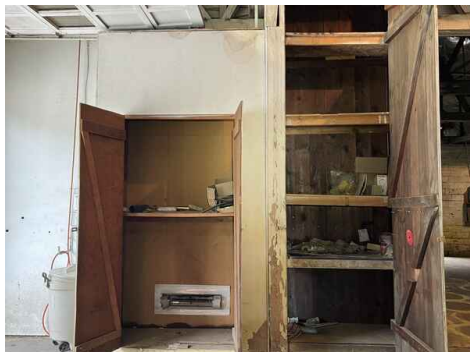
Main Warehouse Space
