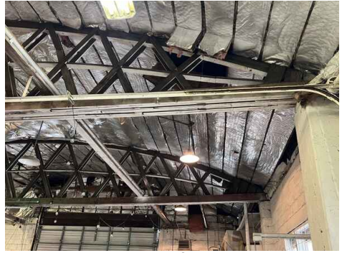
Interior Roof Structure
