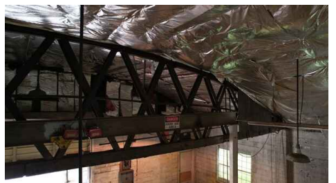
Interior Roof Structure
