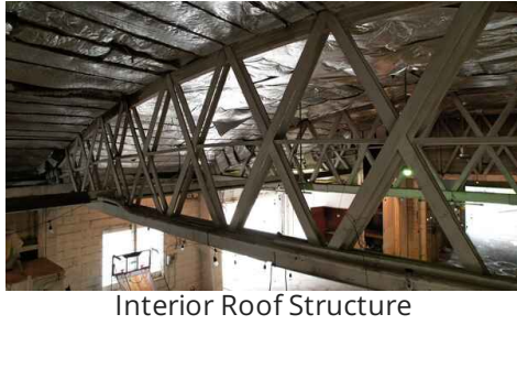
Interior Roof Structure
